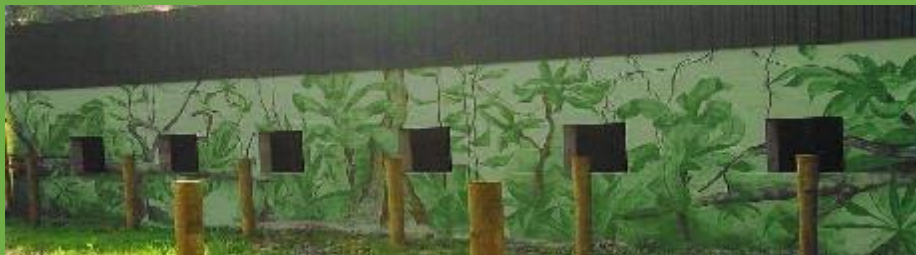
Outside of new primate building. Lea, a T&D's volunteer, painted the beautiful mural. The holes in the wall will be the animal's access to the outside enclosures.
